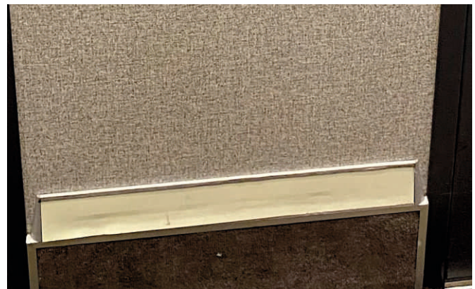
Damaged profile and insert
