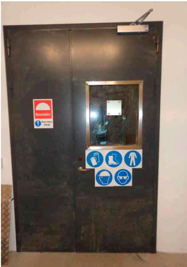
Picture. Safety signs piled up
