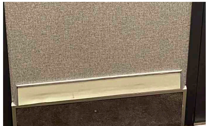
Damaged profile and insert
