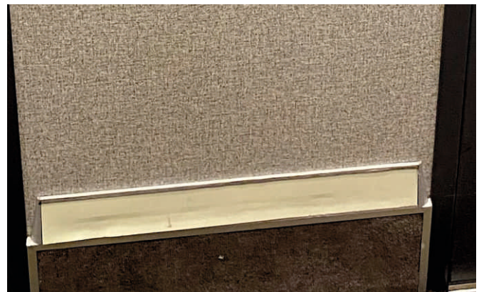
Damaged profile and insert
