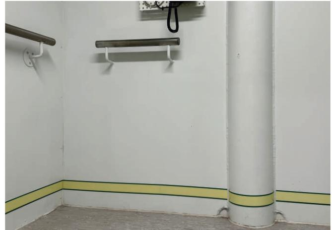
**3L-PL™** strips have a standard length of 1 m, 50 mm height and are produced with the high luminescence class XXL. All strips have a self-adhesive backing for easy fixing during new builds or refurbishment projects. **3L-PL™** strips are besides Non PVC/halogen-free, flame retardant and therefore exceeding all current requirements. Upon request we can manufacture **3L-PL™** strips in other widths and/or with other coloured marking stripes.
