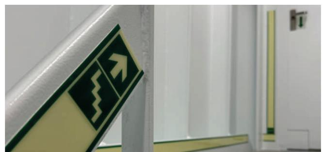
Note; The width of the photoluminescent material in the strips with the green edges is shown in parentheses, the width of the green edges is 2 x 5 mm.
